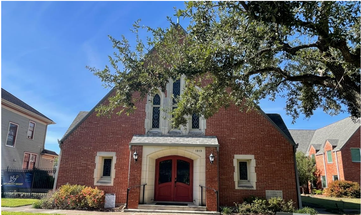
Church Entrance on Heights Blvd.
