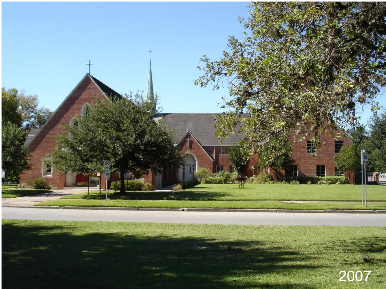
East Elevation, Contributing Original Church circa 1947, from Heights Blvd.
